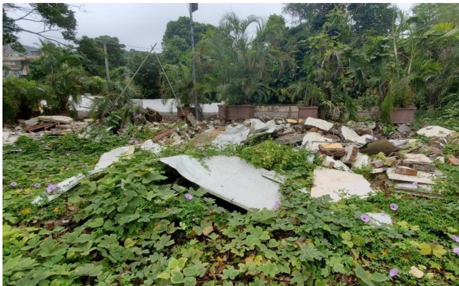
Photo 1.4 Demolished Structures and Construction Waste in Zone 1 (Facing West)
