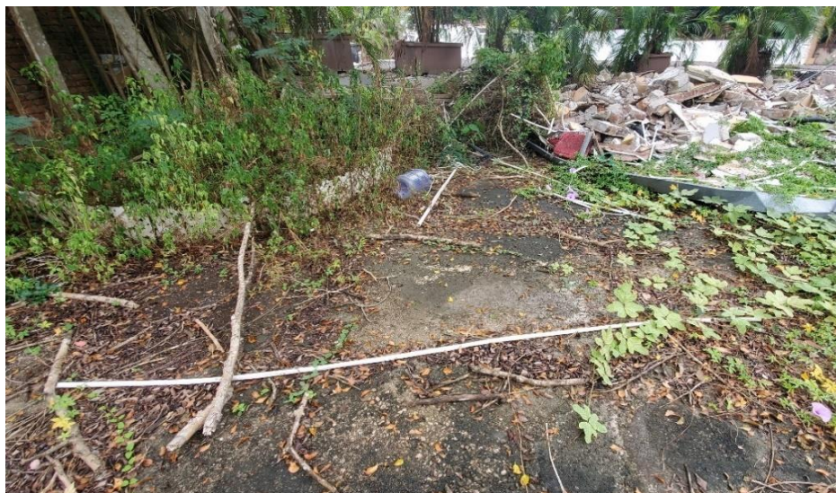
Photo 1.2 Concrete Ground Surface in Zone 1
